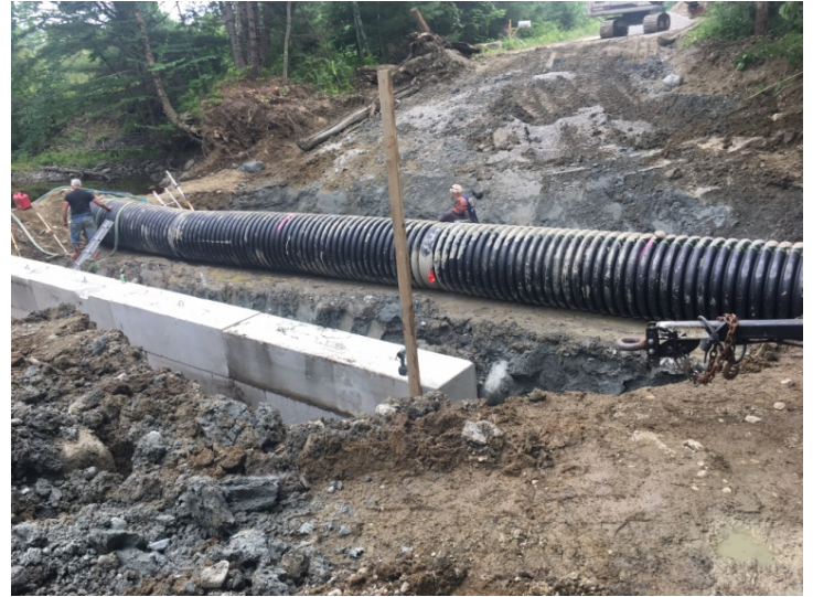
Culvert used as temporary bypass
