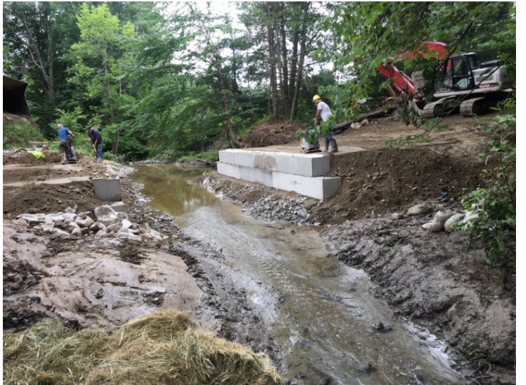
Culvert used as temporary bypass
