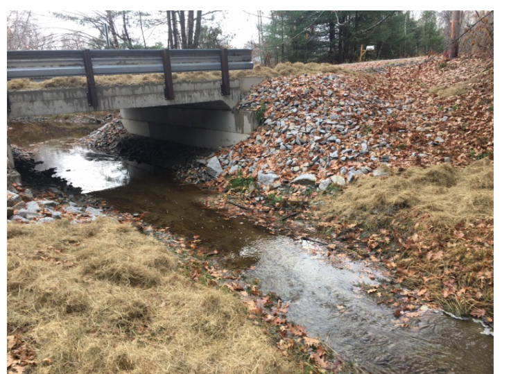
Finished concrete box culvert
